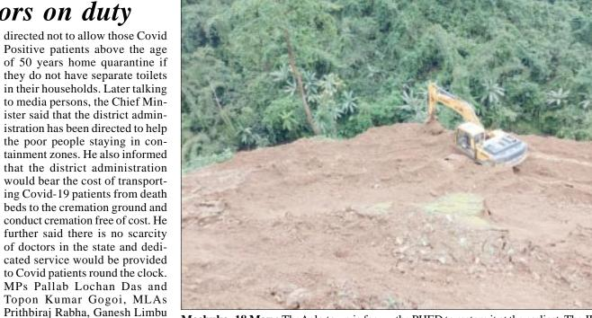
Mechuka, 18 May : TheAalo town is facing acute water supply for the last three days due to extensive damages caused to to 300mm DI Pipe catering water needs of the town. The damage was due to erosion triggered by monsoon. The huge accumulation of sand silts and debris above the in the construction work is also assisting water scarcity problems.
